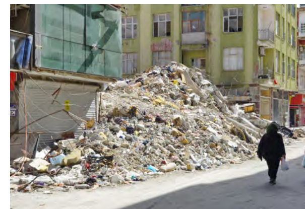
İskenderun, Turkey | March 10, 2023: A man walks by collapsed buildings in southern Turkey nearly a month after the earthquakes struck the region.
